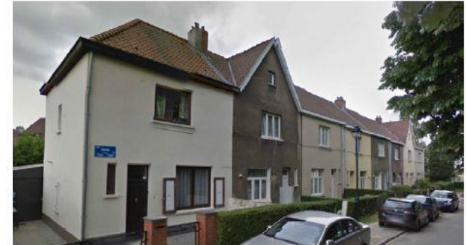
Photo situation existante
